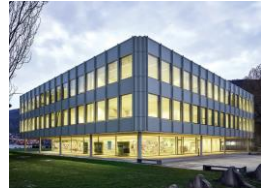
Gymnase Strandboden Bienne
